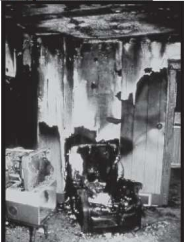
A Typical Conical Fire Pattern
