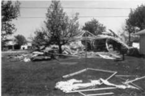
High-Order Damage Shown by Shattered and Splintered Remains of a Four-Bedroom House.
