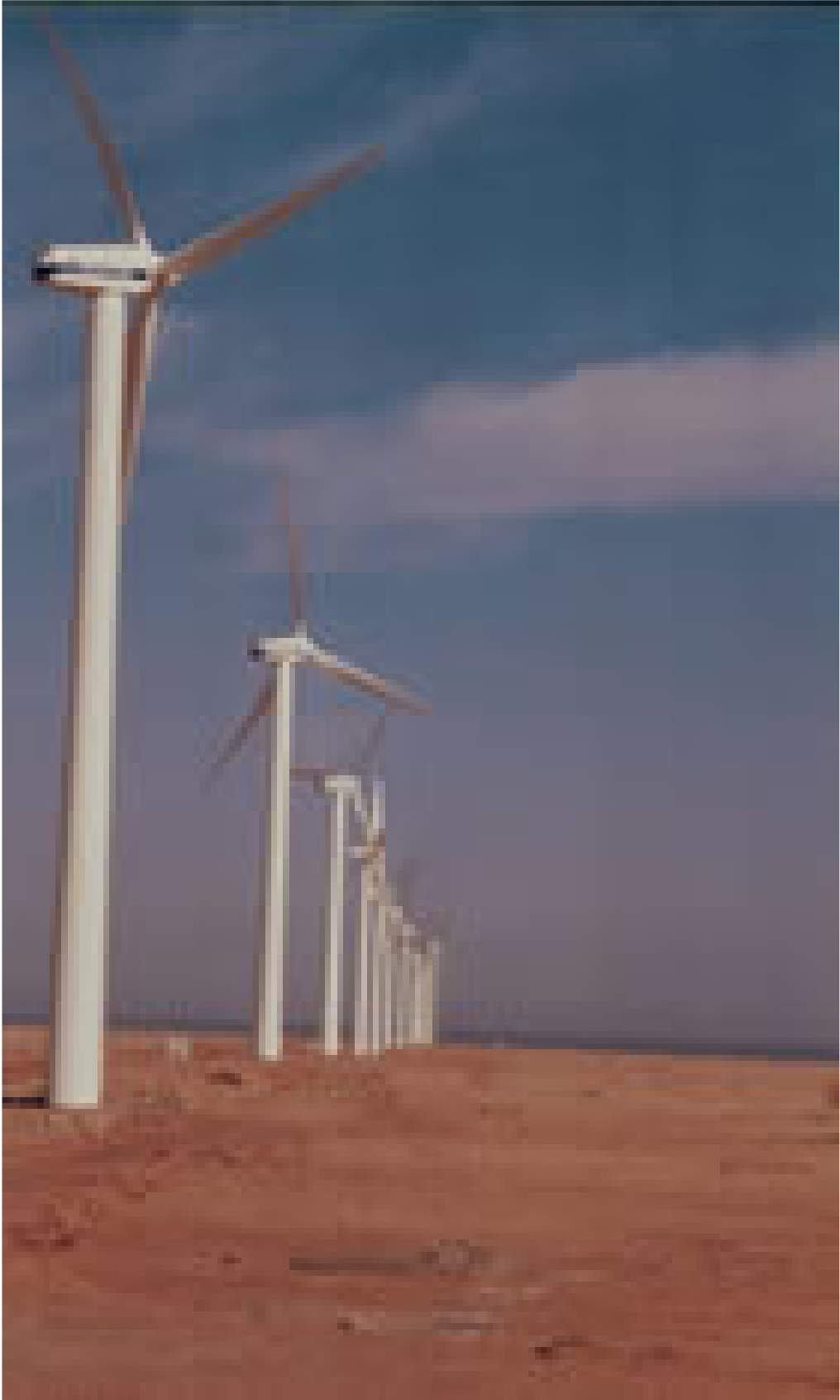
Overview for Zafarana wind farm
