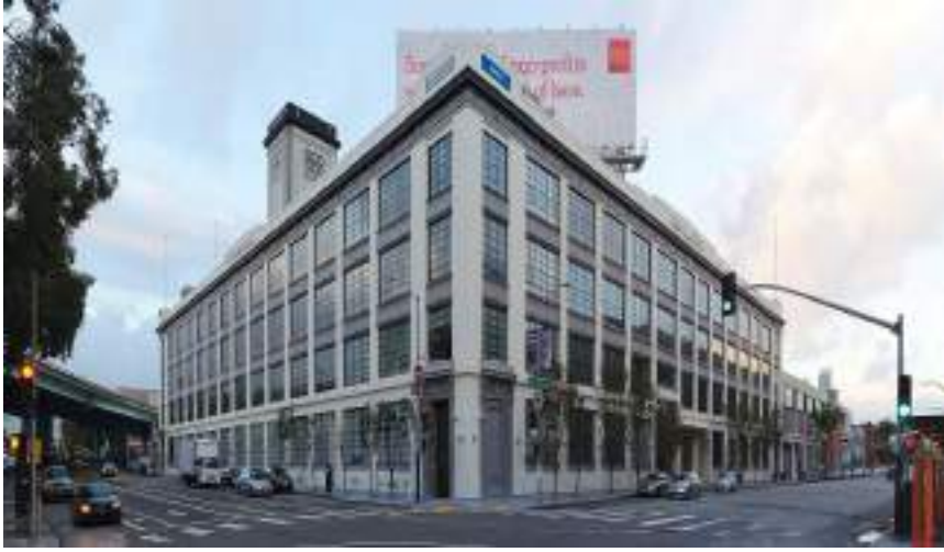
A building in San Francisco. The building contains the Airbnb North American headquarters.
