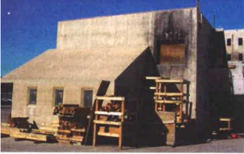
Burn buildings are a great way to teach firefighters about fire dynamics in the modern fire environment, but we must ensure that our live-fire training programs are in compliance with NFPA 1403.
